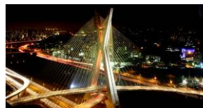
Brazil Infrastructure Paving the Way May 5, 2010
