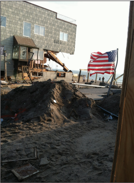
Sea Gate, Brooklyn, a community devastated by the storm.
