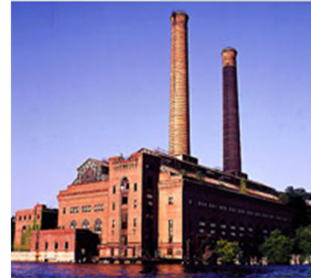
The former Glenwood Power Plant YONKERS, WESTCHESTER COUNTY
