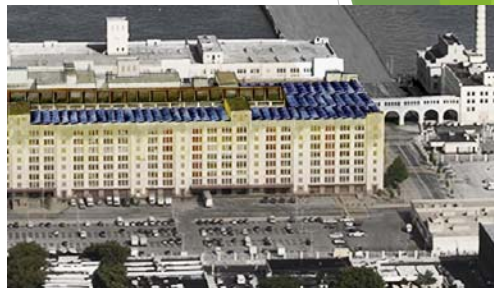
Smart Grid Demonstration Project at Brooklyn Army Terminal combined Solar PV, Battery Storage and building energy management system
