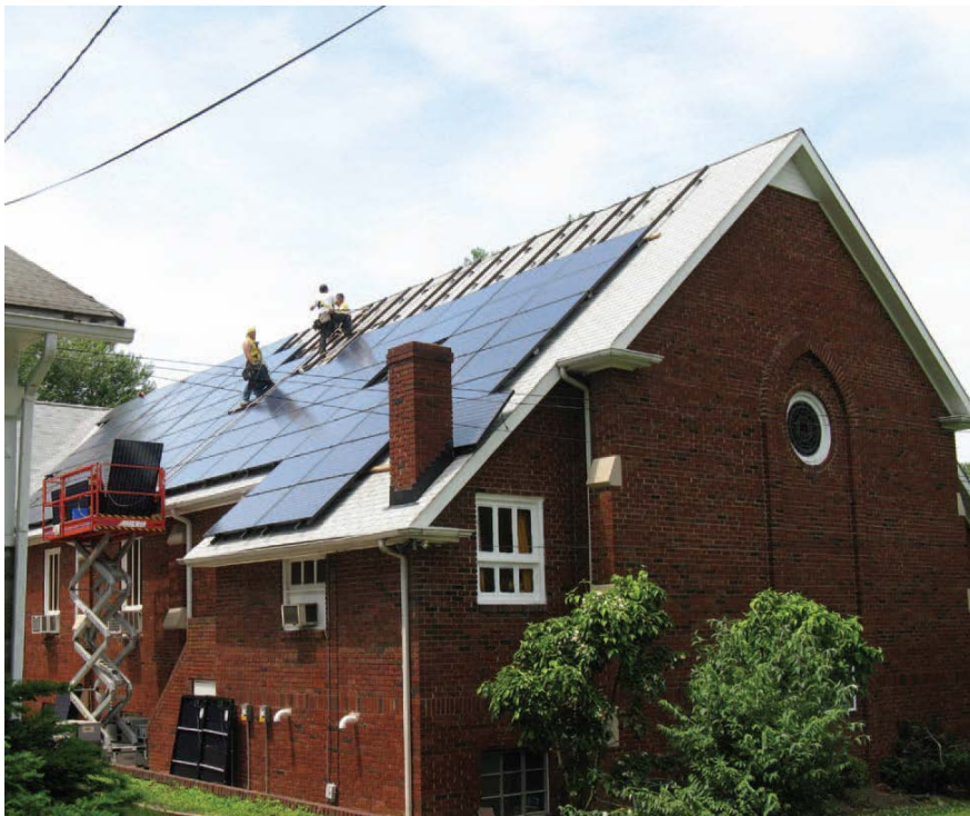
Photo from a Steep Roof, University Park, Maryland
